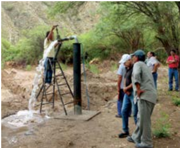
With the municipal administration of Belén, Catamarca, a water well has been developed along the Belén River to maximise drinking water supply.
