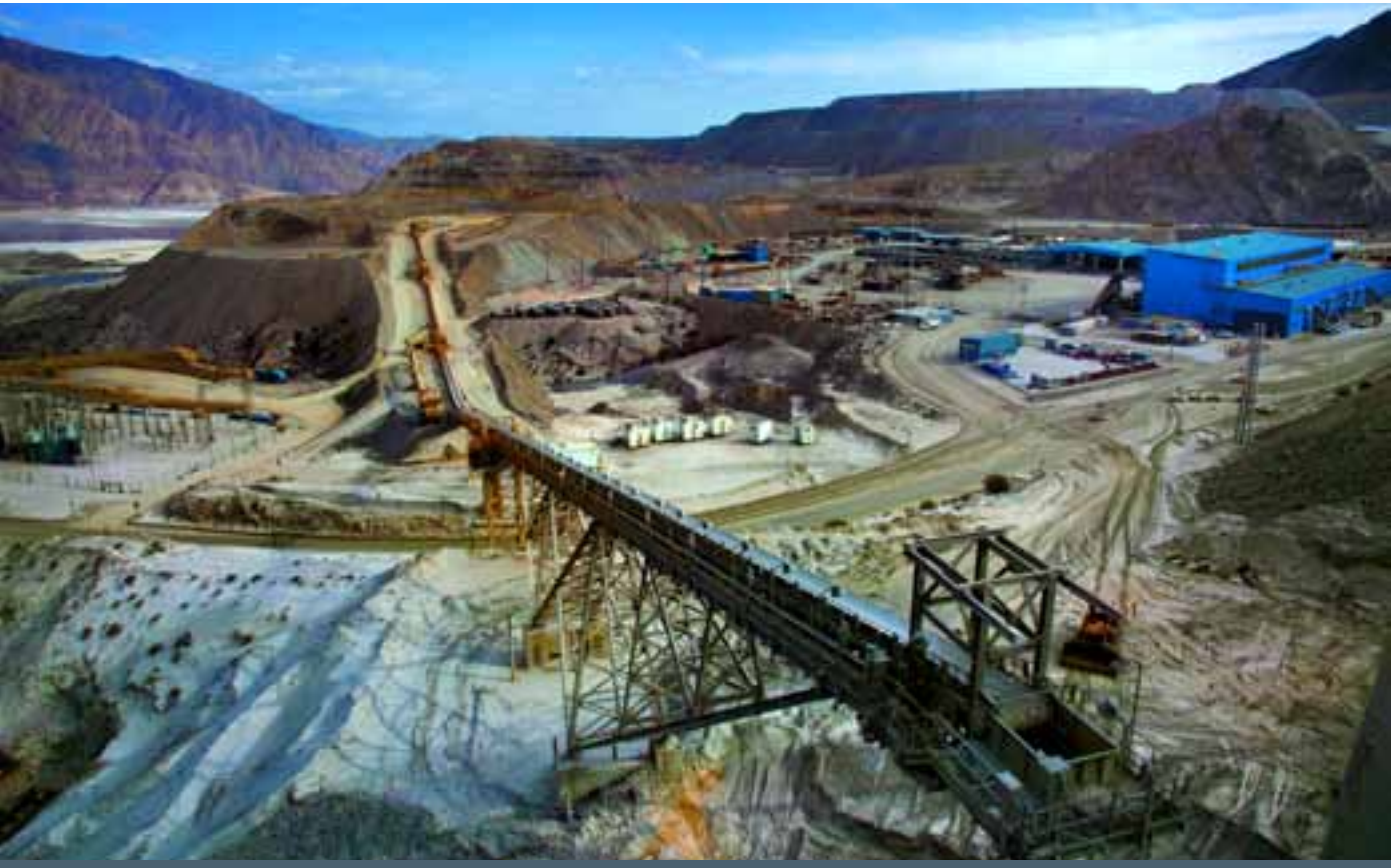
Feeding system that takes milled rock to the stock pile.
