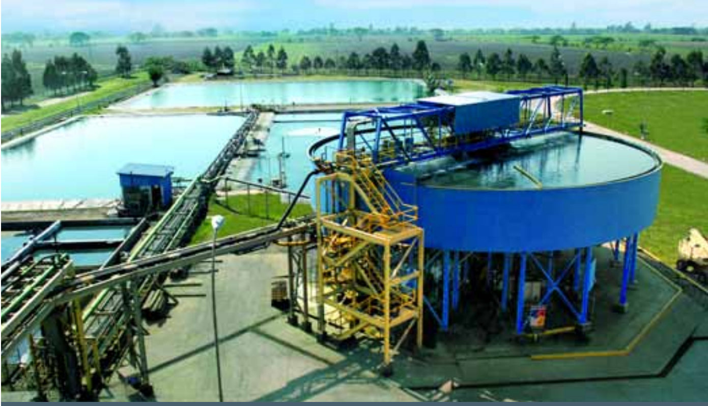
At the Filter Plant, the concentrate is dewatered. Before discharging into DP2, water is purified.
