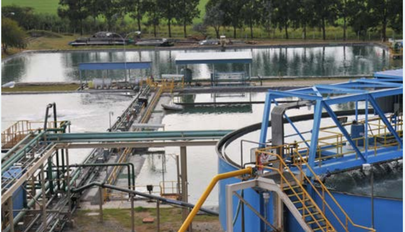
At the Filter Plant located in Tucumán, concentrate is dewatered and water is tested in accordance with provincial regulations.
