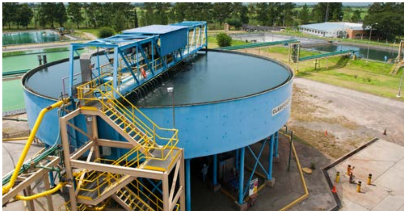
Tucumán's Filter Plant where concentrate is dewatered to reach a 7% humidity level.
