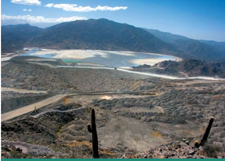
Water from the tailings dam is pumped back to the process.
