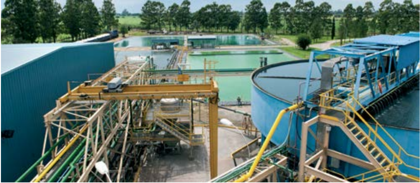
Filter Plant in Tucumán where concentrate is dewatered and water is treated.
