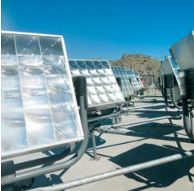
Solar energy generation pilot plant at the mine site that generates 3 kW. We are considering building a similar plant in nearby towns.
